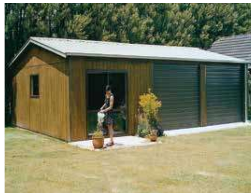
9.6m x 6m Double Garage with a Sleep Out. Clad with 12mm Shadowclad plywood, with matching tilt doors and joinery.
